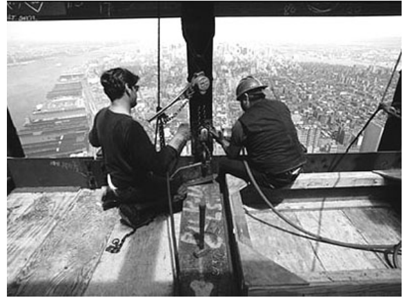
Figure 12 View of Floor and Exterior Wall System from within the building [15]
